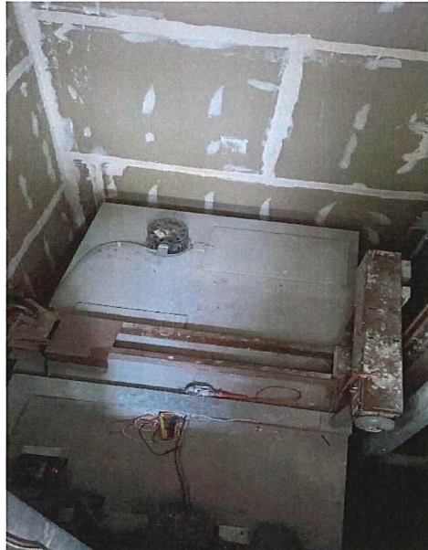
Existing Hydraulic Elevator – Car / Hoistway
